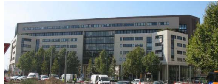
Building A view
