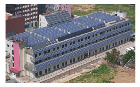
360kW solar cooling system with heat pipe solar collectors, Sanpu company Office building, Beijing
