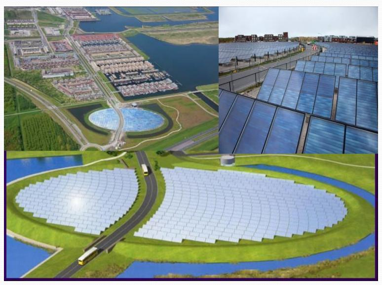
Flat Plate Collectors 7000 m<sup>2</sup> Production 10,000 GJ/y at 75 C
