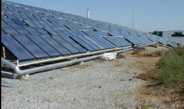
Air-conditioning of a production hall in Greece
