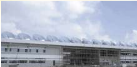
A typical solar installation
