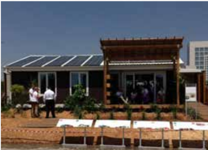
3 rd build at competition site
