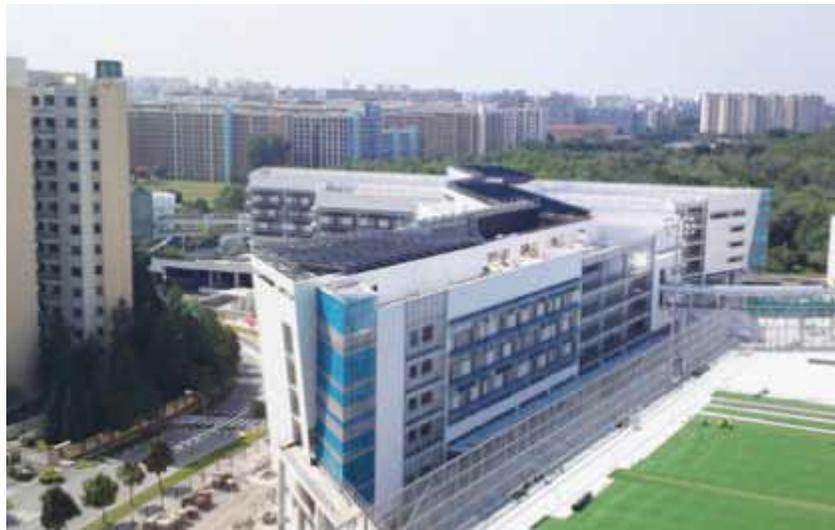
United World College in Singapore, 3900 m<sup>2</sup> solar collectors on the roof, delivering 2200 MWh per year and providing a cooling power of 1.5 MW. Heat is converted into cooling by an absorption chiller.
