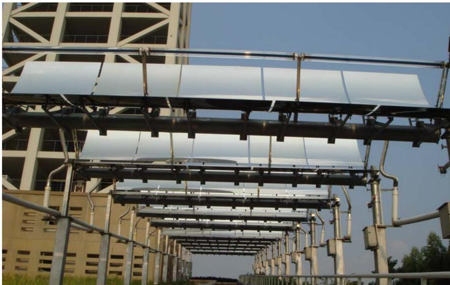
**Figure 20: Installation of parabolic collectors on the ground besides the building (Source: SJTU)**
