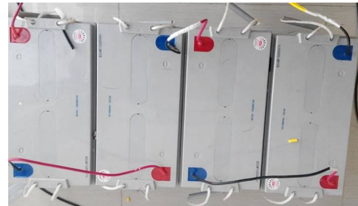
The storage battery
