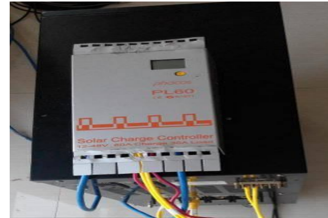
The control inverter
