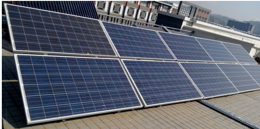
Photovoltaic generate electricity components
