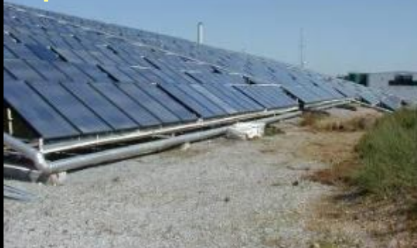
Air-conditioning of a production hall in Greece
