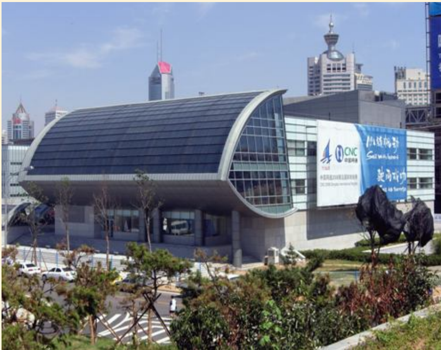
Olympic Sailing Village, China: Solar cooling
