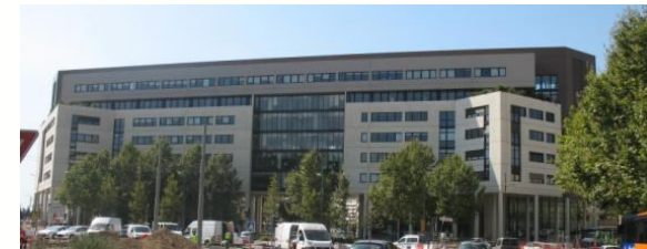
Building A view
