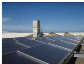
Solar cooling installation for a Tertiary building in Tropical climate (Source : TECSOL)
