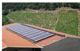
Solar cooling installation for a wine cellar in South of France (Source : TECSOL)
